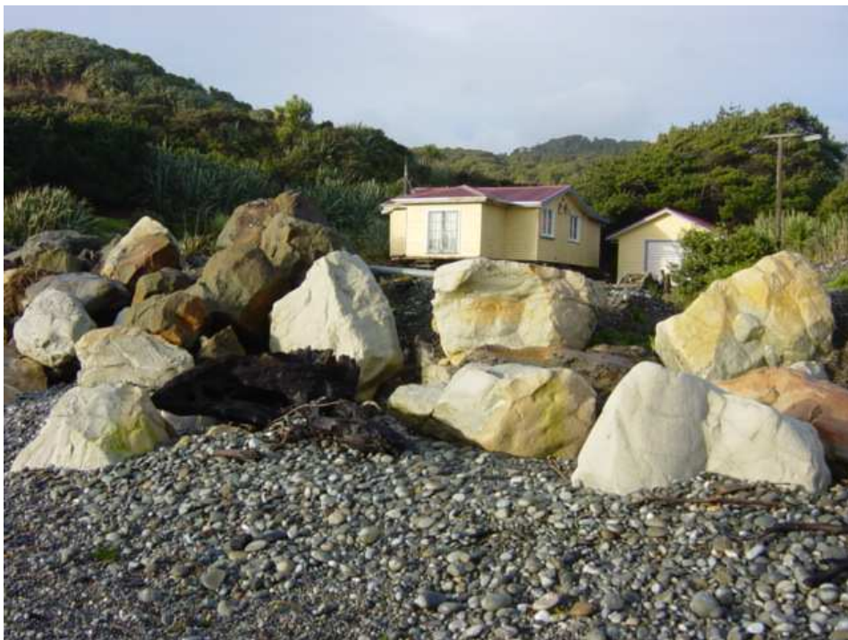
Figure 7.0 Photograph displaying the Forbes property and riprap revetments 24/6/07
